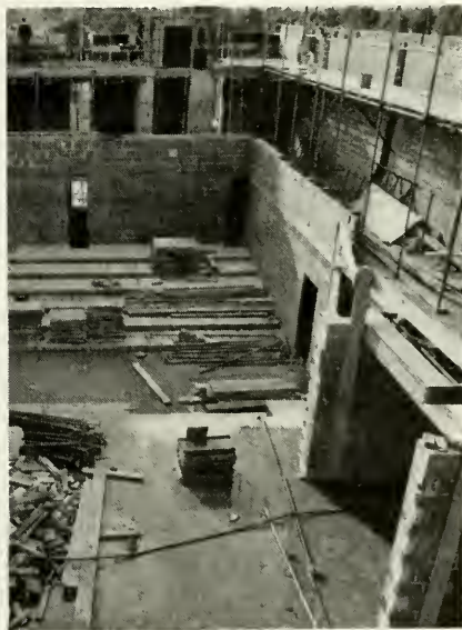
Interior construction, September, 1957
